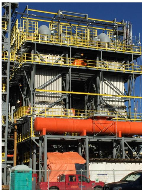
Installation of primary and secondary acid mist WESP trains for acid plant gas cleaning
