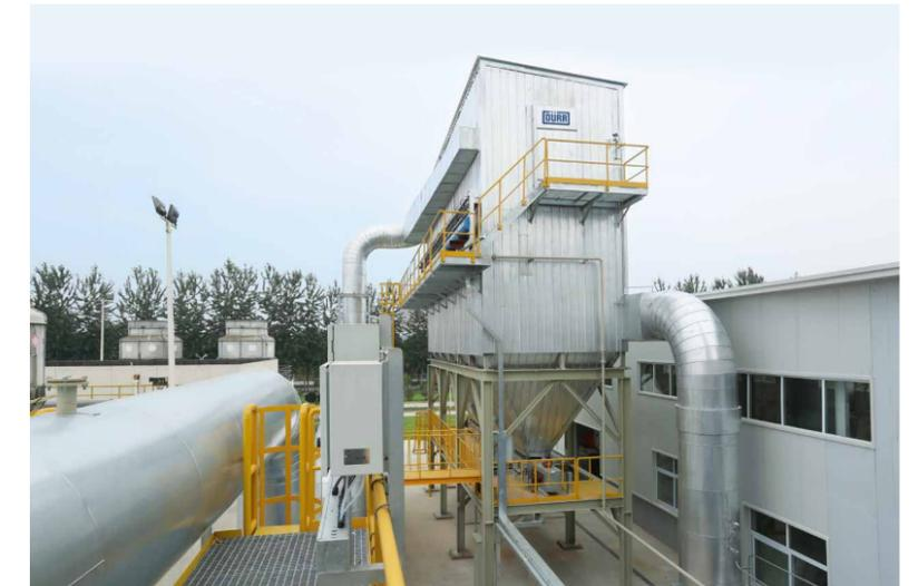
Catalytic candle filter for simultaneous reduction of pollutants.
