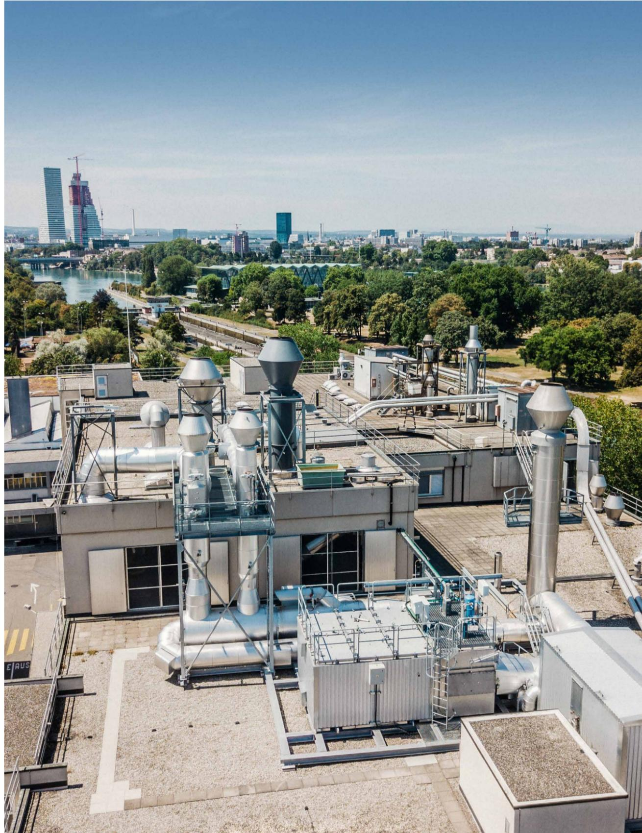
Flameless regenerative thermal oxidizer Oxi.X RV powered by renewable energy sources.
