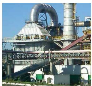
Particleboard dryer wet ESP system
