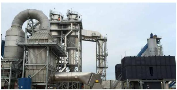
Wet electrostatic precipitator
