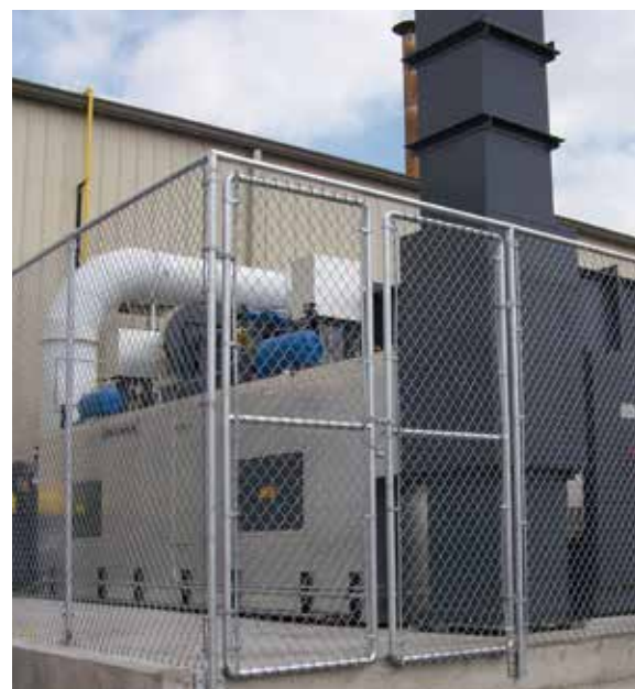
The MILLENNIUM RTO has a small footprint, which allows the unit to be installed in tight spaces.
