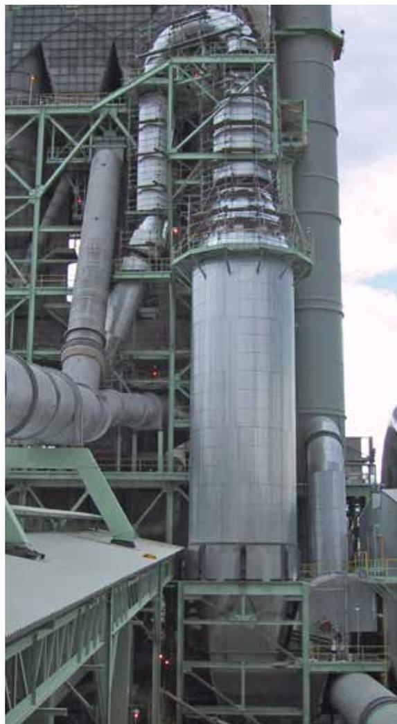
Evaporative gas cooling and conditioning tower
