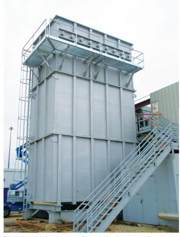
Dürr Universal designed and manufactured this exhaust system for a Westinghouse 251 gas turbine power generation peaker unit. The original unit experienced significant deterioration to the inside liner sheets and exhaust baffles.
